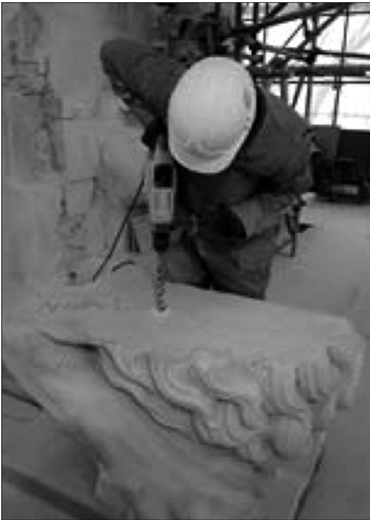
Drilling hole for Lewis pins.
