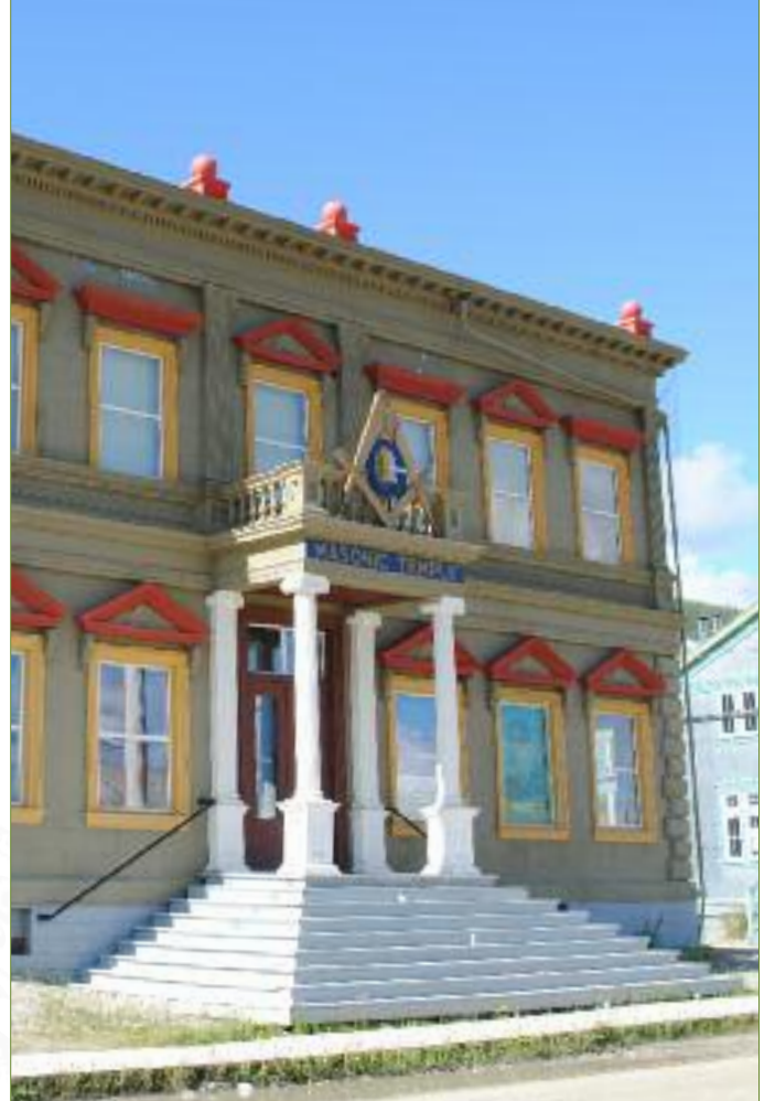
The home of Yukon Lodge 45 in Dawson City recently enjoyed a facelift.
