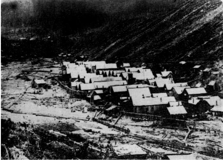
"The morn' was bright and clear — a hard frost was on the sluice boxes."
